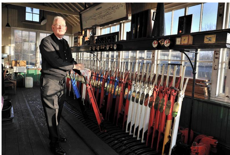
Traditional signalling equipment protects the safety of the line at Loughborough (Photo: GCR)
